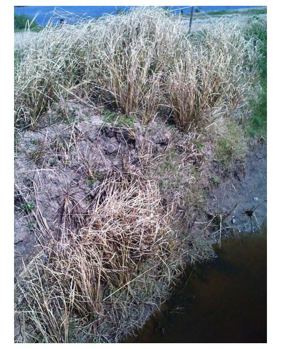
the bottom row of Vetiver, slid down because the bank sheared off. The bank is very steep here, going down to a depth of about 2 meters
